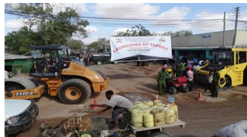
Figure 2: Ongoing road works in Garisa County
