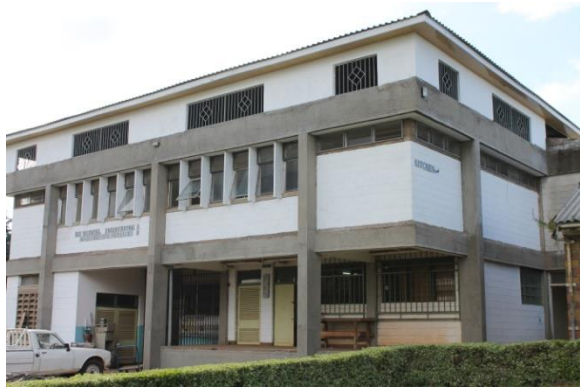
Nyamira Referral Hospital undergoing renovation
